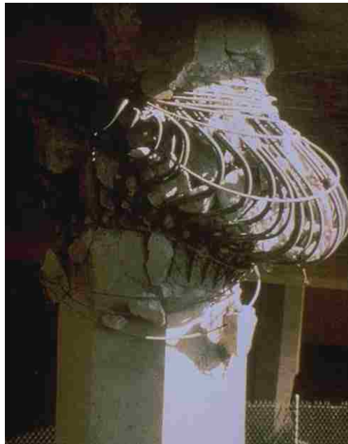
Figure 2.5: Inadequate confinement in the I-10 La Cienega-Venice overpass led to buckling of longitudinal reinforcement and crushing to core concrete during the 1994 Northridge earthquake [18].
